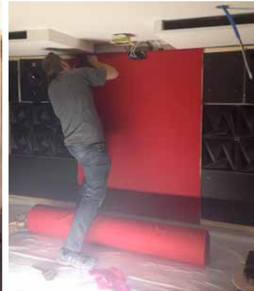
**CATS** is designed to be extremely straight forward to install. It should be mounted directly to the wall with appropriate screws. Most acoustically isolated walls are constructed such that no special wall fixings are required to secure the panels.
